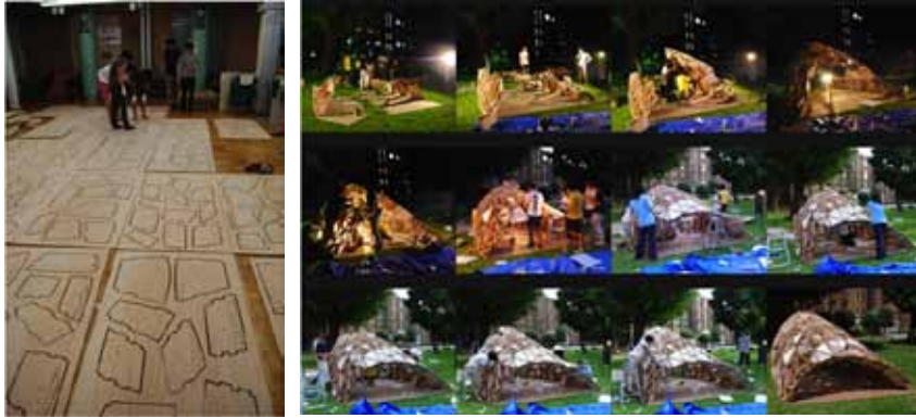
Figure 8 (left). Plywood panels ready for assembly. Figure 9 (right). Assembly process.
