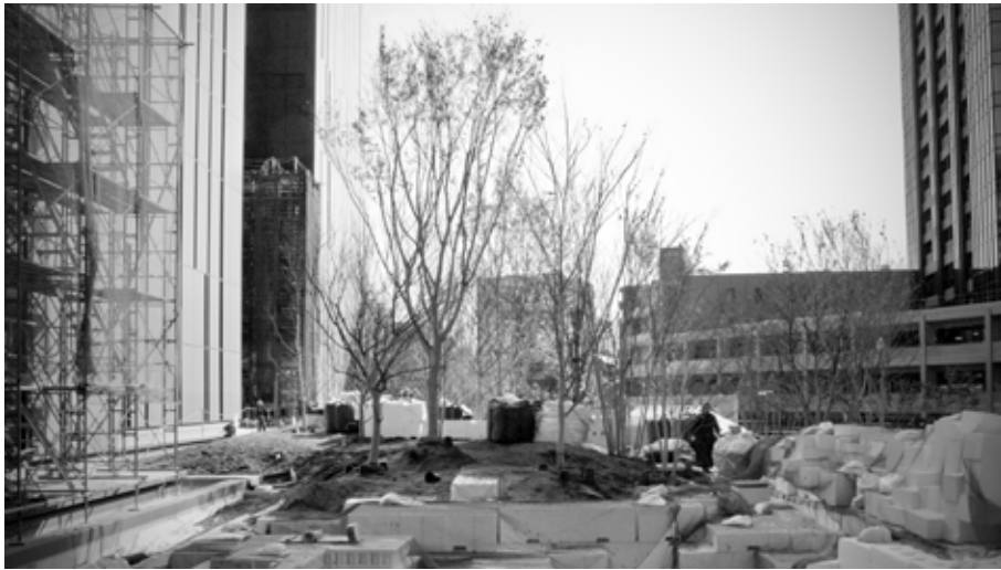
Figure 6. The SONY forest in the urban context (The construction site on Nov.19 th , 2010).
