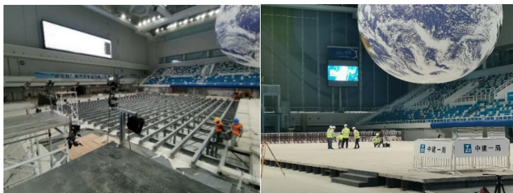
Figure 2. Application of a DfD-based fast-built steel structure system in the ice-to-water conversion system for the Olympic curling Hall in the Chinese National Aquatics Centre("Water-Cube")
