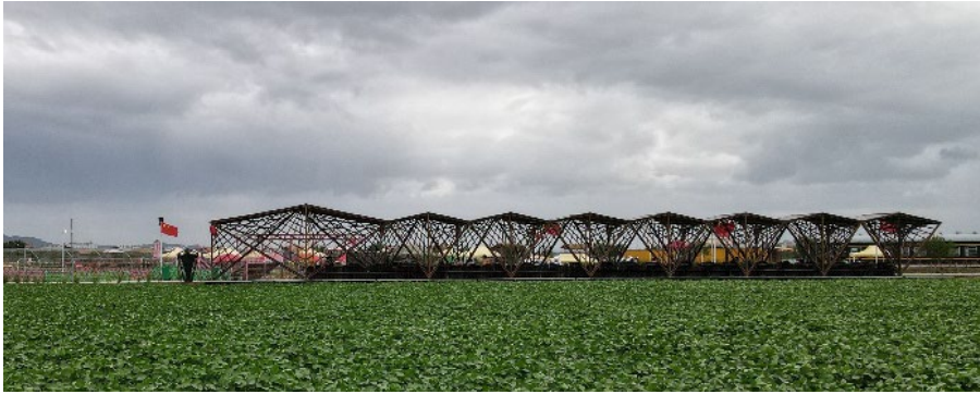
Figure. 1. The bamboo pavilion "Diecui Gallery"
