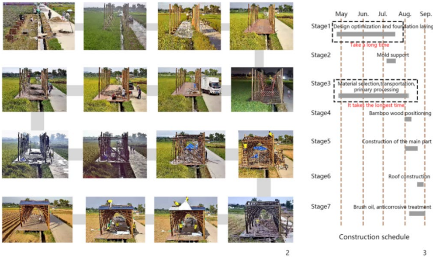
Figure. 2&3. Construction process and schedule
