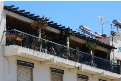
Figure 2 Balcony in Távira (Portugal)
