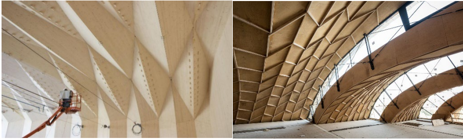
Figure 1. Two examples of IATPS: the theatre of Vidy in Lausanne (left, © Ilka Kramer) and the multipurpose hall of Annen in Manternach (right, © Valentin Bianchi).
