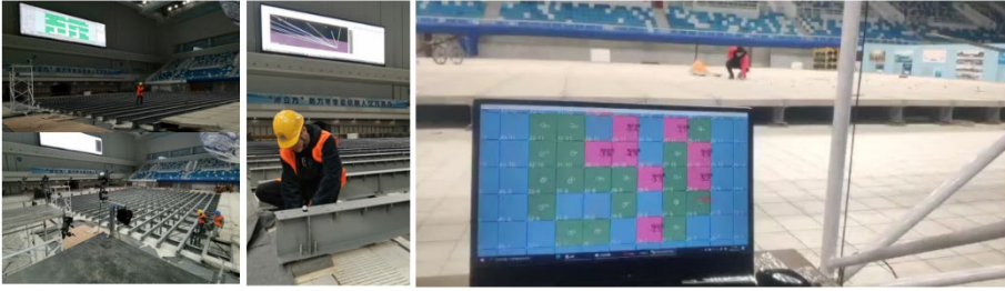
Figure 10. On-site application of the tuneable structures with the mocap beacon and the levelling support system
