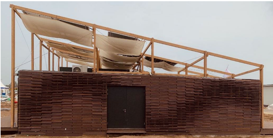
Figure 2. The use of laminated bamboo material in Aurora's façade
