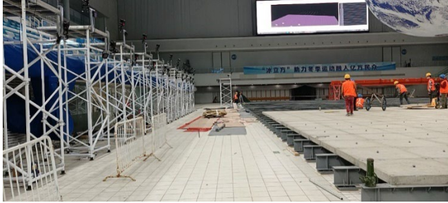
Figure 5. Construction site and the arrangement of the sensors
