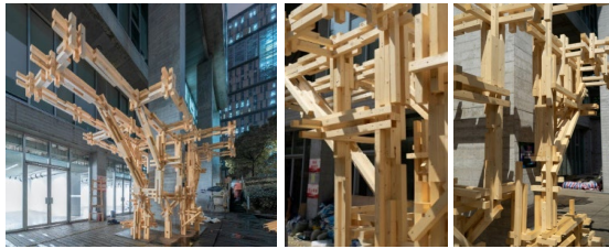
Figure 8 Robotic fabricated Spatial Glulam Structure
