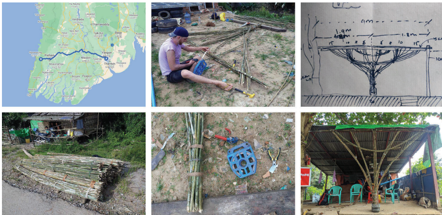
Figure 5. Mockup prototype as a structural column for a shelter in Yankin Township by Blue Temple Co., Ltd.
