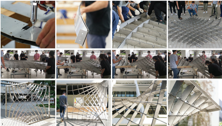
Figure 6. A-D: Prefabrication. E-H: Elastic formation. I-L: Completed module.
