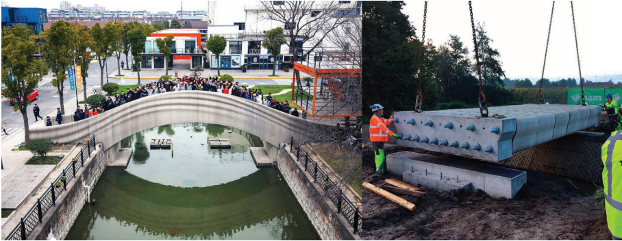
Figure 1. 3D concrete printed arch bridge by Tsinghua University 2019 (left) 3D concrete printed prestressed bridge by TU Eindhoven 2018 (right).
