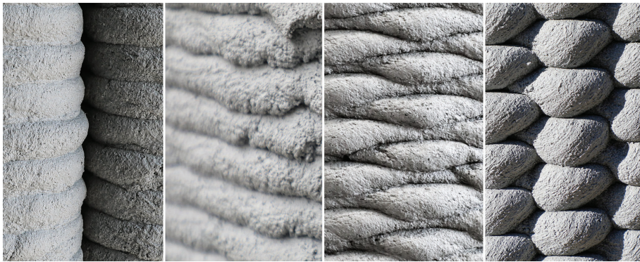
Figure 5. Details of patterns from the C3DP columns designed through toolpath manipulation.
