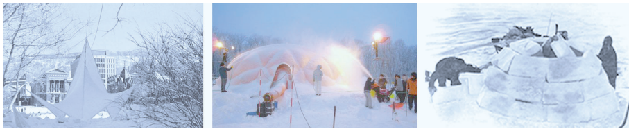
Figure 1. (a) Water sprayed on stretched double-curved subsurface (Sijpkens 2009). (b) Application of snow and water (Kokawa 2012). (c) Igloo under construction (Masterson 2009).
