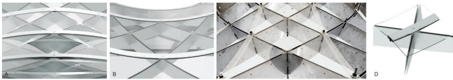
Figure 9. Developable strip facade along the principal curvature directions.
