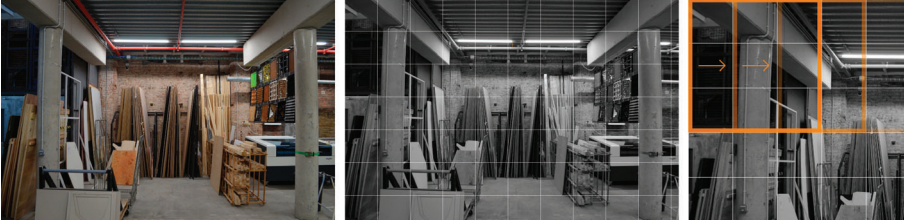
Figure 1. Images from the building inspection analyzed by Larger Sliding Kernel.
