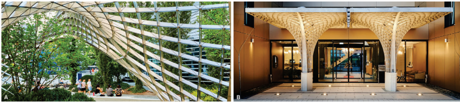
Figure 1. Asymptotic lamella gridshells. A: The Inside/Out Pavilion at the Technical University in Munich. B: The Intergroup Hotel Canopy in Ingolstadt.
