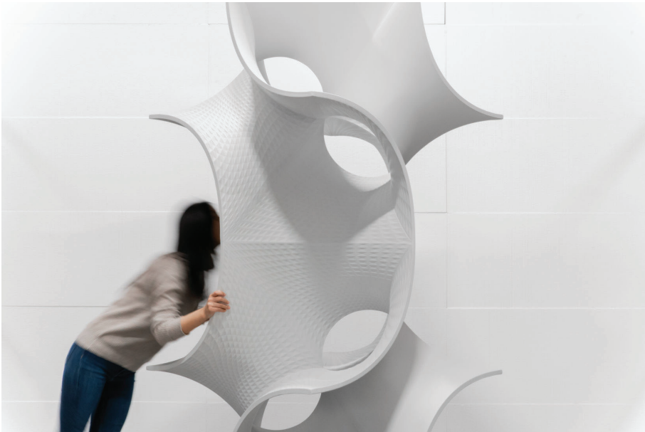
Figure 6. Min Max Structure as exhibited in Swissbau. An 18mm thin shell structure standing 2 meters high with minimal use of material (overall only 80 liters (40 per unit) of GFRC was used).
