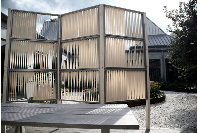
Figure 7. Physical demonstrator placed in an outdoor environment. The façade system clearly displays its environmental performance towards shading the sun and directing views.
