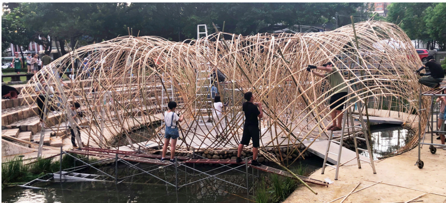
Figure 5. Under construction: grid densification.
